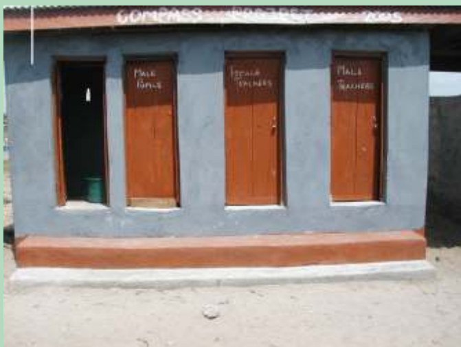
New toilet facility in Folu Community Primary School compound Photo: Morris Kamara, COMPASS Lagos
