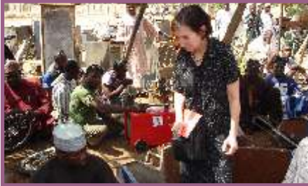
Hope Sukin observing KPVTA welders using USAID-funded welding equipment Photo: Bala Manaseh, COMPASS ACO
